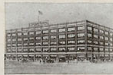
Omaha, Neb. 5 stories 284 x 120—170,400 square feet floor space
