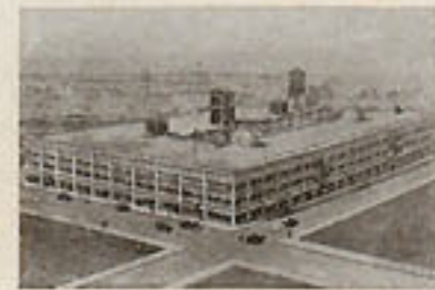
Kansas City, Mo. 3 stories 421 x 251—317,013 square feet floor space
