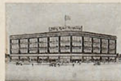
Louisville, Ky. 4 stories 206 x 100—82,400 square feet floor space
