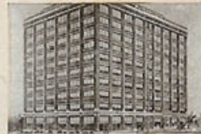
Minneapolis, Minn. 10 stories 198 x 145—287,100 square feet floor space
