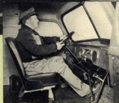
Seats are scientifically designed for driver comfort, and adjustable to the driver's size. Front compartment is unobstructed—levers are relocated to permit easy entrance or exit from either side.
