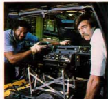
Instrument panel installation.
