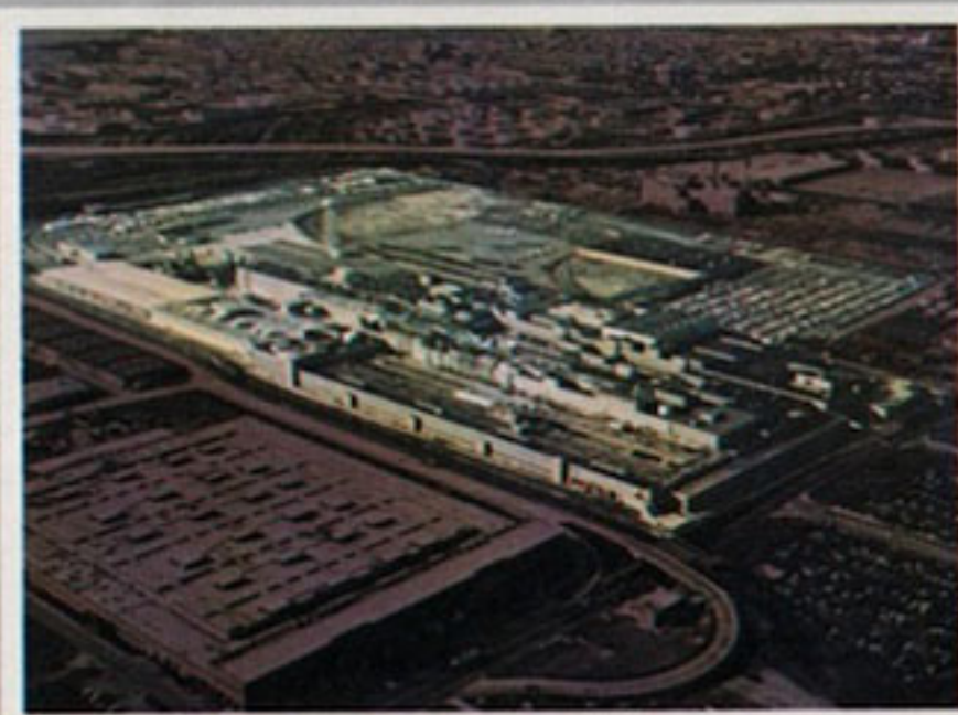
GM Van Plant in Baltimore, Md.
