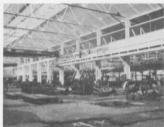
Conversion: tearing down fixtures and machines—typical of the change-over from peace to war production
