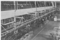
"Suspended assembly" at the new Flint plant
