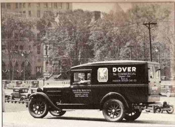
1929 ESSEX--In 1929, Hudson Motor Car Co. introduced a series of Dover commercial vehicles. Body types included a panel delivery, a canopy express, an open express and a screen-side express. Wheelbase was 110-1/2 in.
