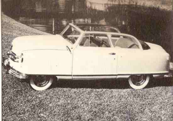
1950 NASH Rambler, Model 5021--This 100-inch-wheelbase convertible is a historic vehicle: the first compact car, introduced in March, 1950. In naming it, Nash Motors revived the historic Rambler name. With a peppy 82-horsepower six-cylinder engine, it gave 25 to 30 miles per gallon of fuel.
