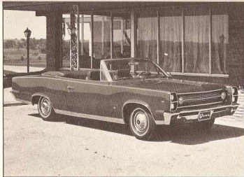
1967 AMBASSADOR DPL, Model 6787-7--A handsome two-door convertible was added to the DPL series in 1967. A new top mechanism, also standard on the Rebel SST convertible, folded flush with the body line.
