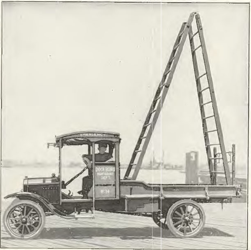
Emergency Truck operated by Dock Board Maintenance Dept., New Orleans, La.
