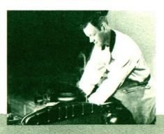
The power cylinder is now located right at the steering link. Here the cylinder can intercept road shocks and smother them before they ever get to the steering gear and column. And having the cylinder right where the steering is done means more positive action.
