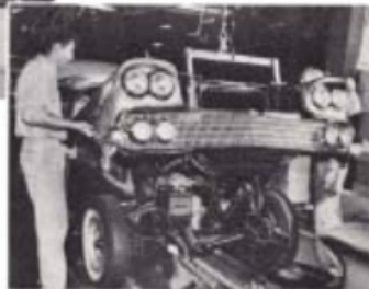
Front fenders and grille drop into position as a unit.
