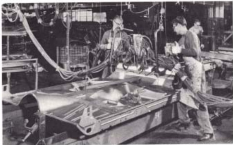
The famous Body by Fisher begins with the pan—or floor—of the car.
