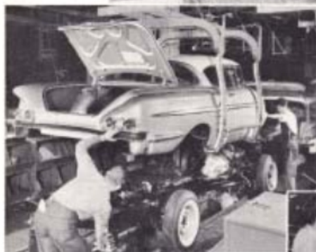
The body meets the chassis at this point.
