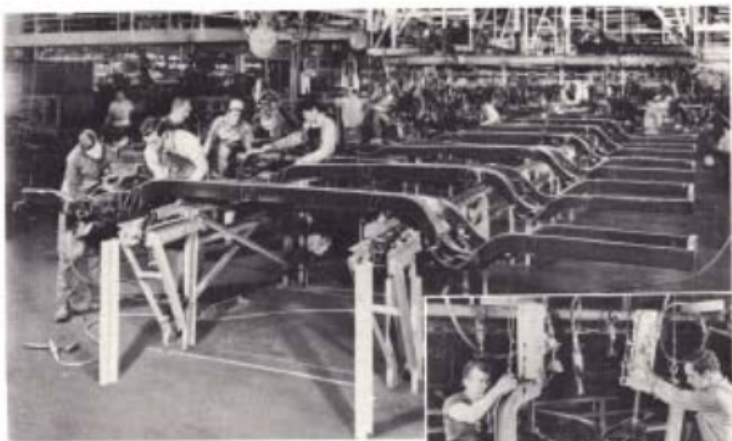
Assembly operations begin with the frame in an upside-down position.
