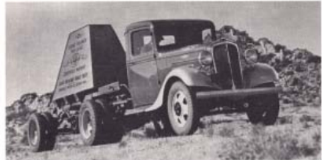
Chevrolet trucks demonstrated outstanding economy in a series of AAA tests in 1936. This 1 1/2-ton truck is hauling a trailer with a 5-ton load up Pikes Peak. Another typical test was the coast-to-coast economy run from Los Angeles to New York carrying the same load.
