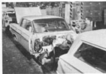
Adjacent Fisher Body plant delivers bodies to Chevrolet assembly line. Workmen ready the body for "body drop" operation.
