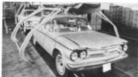
Cradle carrying Corvair is automatically released on moving flat-top conveyor.
