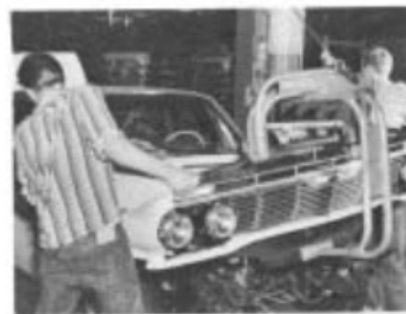
Body meets chassis. Workmen secure body to chassis. Rear deck remains up for other assembly operations.
