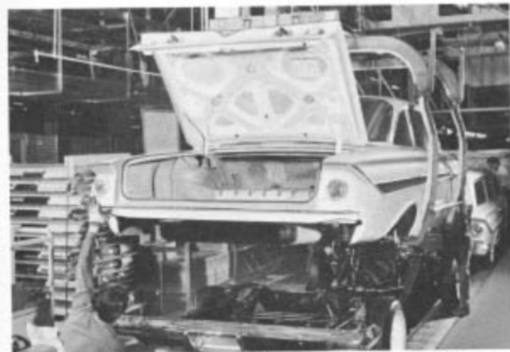
Body meets chassis. Workmen secure body to chassis. Rear deck remains up for other assembly operations.
