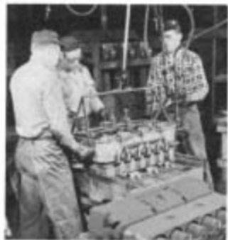
Removing cylinder block casting from sand mold.
