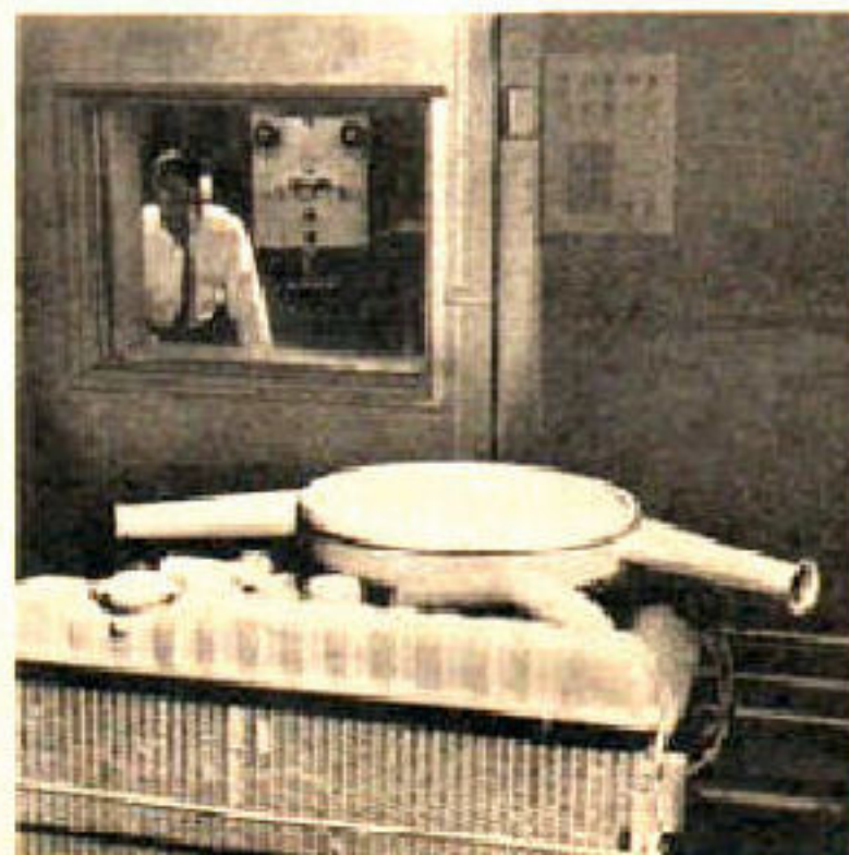
Ninety below! Toronado Rocket V-8 was started, stopped, started over and over in Oldsmobile's Cold Room at temperatures as low as ninety below!
