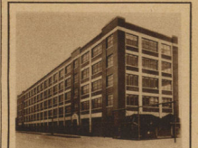
WHERE ALL CHRYSLER CARS have their inception—the Chrysler Engineering Building at Highland Park, Michigan. Five stories equipped with the most modern machinery for research, designing and testing. A staff of approximately 1200 men is employed in this building.
