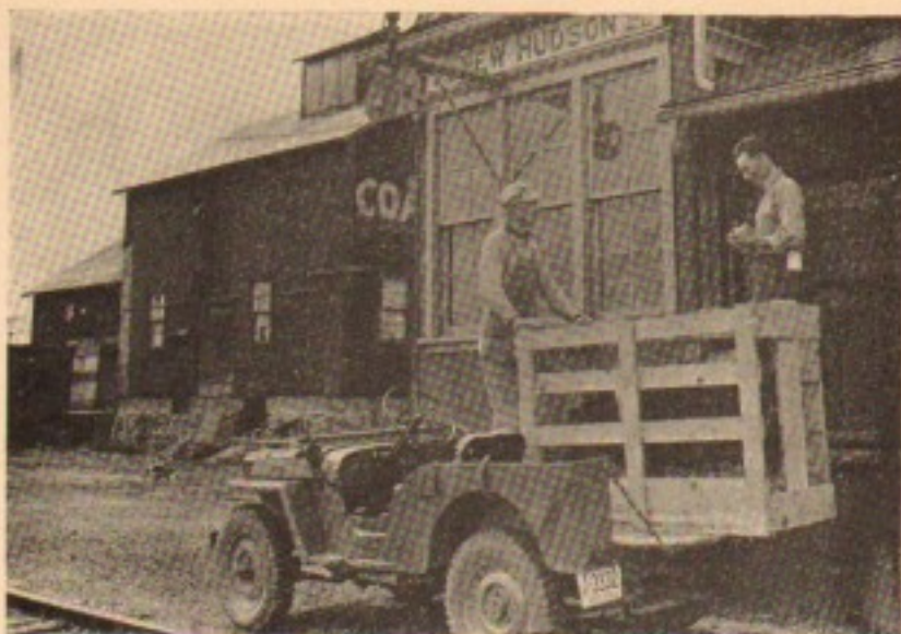
Performing four-fold duty as a tractor, light truck, mobile power unit and passenger conveyance, the Universal Jeep is pictured here picking up freight at the station.
