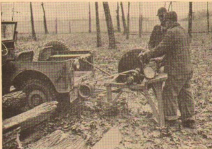
The Jeep with its handy power take-off does a quick and efficient job buzzing wood. Its four-wheel drive and great mobility enables it to carry power to the job over rough terrain.
