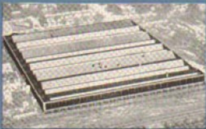
New plant of Nash Motors of Canada, Toronto, Ontario.
