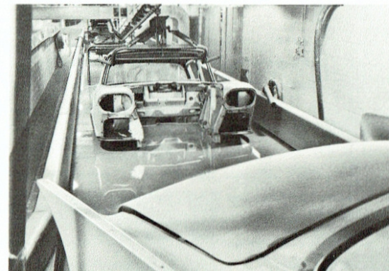
Every Ambassador body-frame structure is submerged in a 15,000 gallon tank of chromate paint primer to protect even the hidden areas against rust and corrosion. Ordinary "spray-on" methods used on most other cars cannot reach these nooks and crannies.
