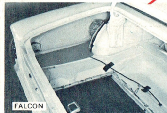
FALCON Check Falcon and Rambler American trunk floor construction. The former uses separate fiber-board inserts at the side, and trunk floor is formed by gas tank (removed).
