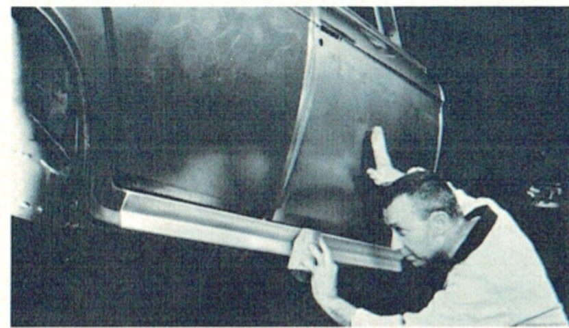
To further protect against rust and corrosion, Rambler rocker panels are galvanized (zinc-clad steel). Here, panels are chemically treated to assure bonding of paint primer.
